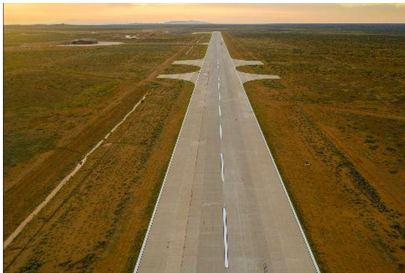
TAKE A 360 TOUR OF SPACEPORT AMERICAN'S FACILITIES
