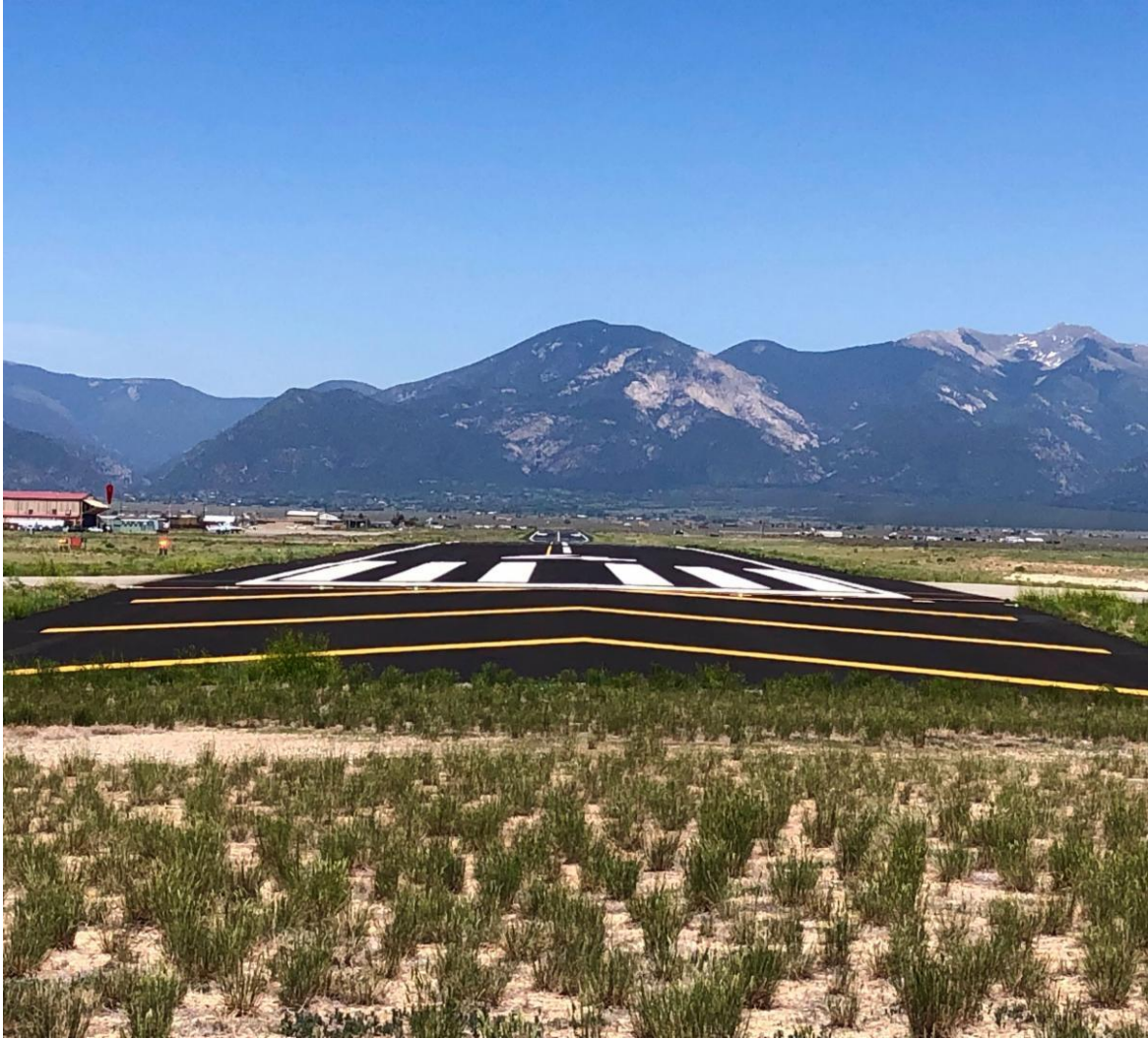
Taos Regional Airport
