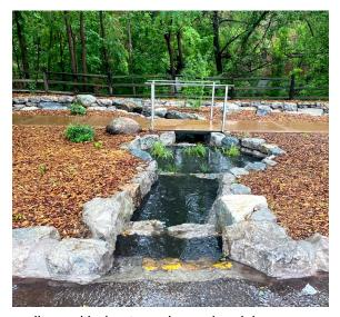
engineered basins significantly improves water quality and helps to recharge low-lying aquifers. The stilling basins upstream at Camino Escondido work to dissipate energy as storm flows enter the Santa Fe River, thereby reducing erosion and decreasing sediment loads entering the river.
