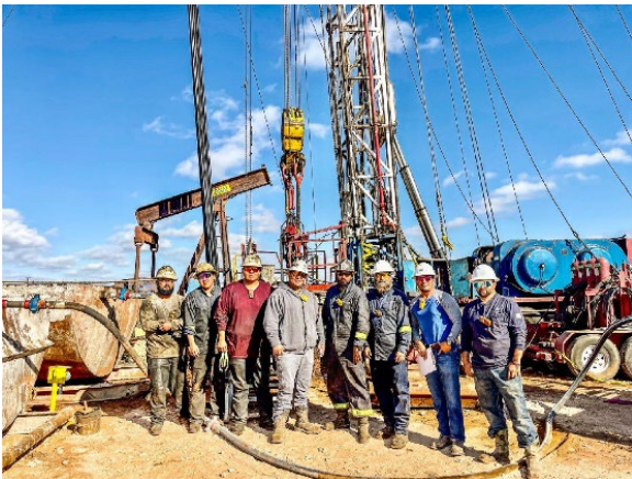
Plugging crew with an orphan well.
