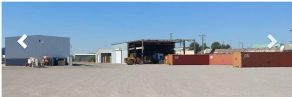
The Big Tuna Pipe property at 1846 W. Amador Ave. includes 13 acres. BULLETIN PHOTOS BY MIKE COOK
