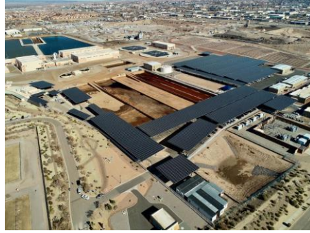
Drone shot of Albuquerque Bernalillo County Water Utility Authority project completed in 2020
