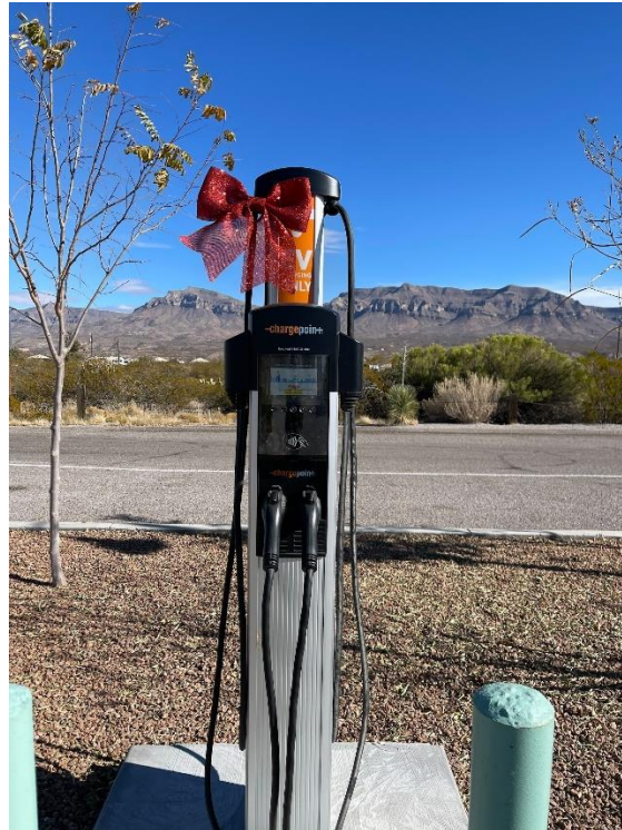
New electric vehicle (EV) charging station at Caballo Lake State Park.
