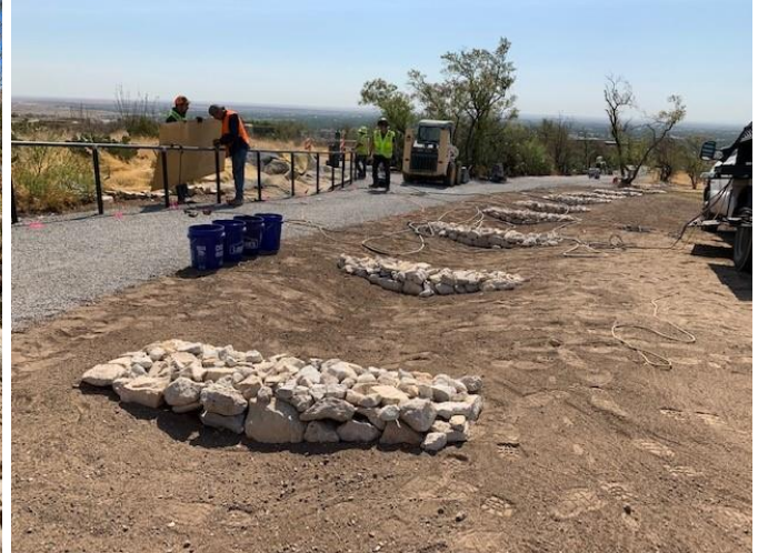
(Figure 1) Workers install new handrailing. (Figure 2) Check dams installed across the swale will assist with slowing water runoff and erosion control. Photos courtesy of NM State Parks.
