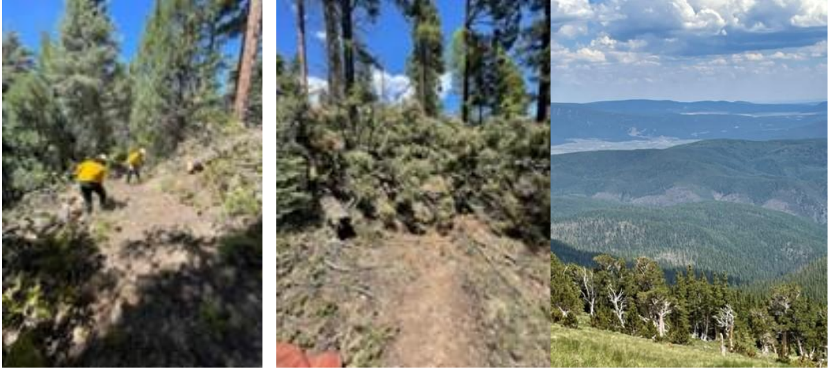
Taos Pueblo Trail Projects, courtesy of Taos Pueblo
